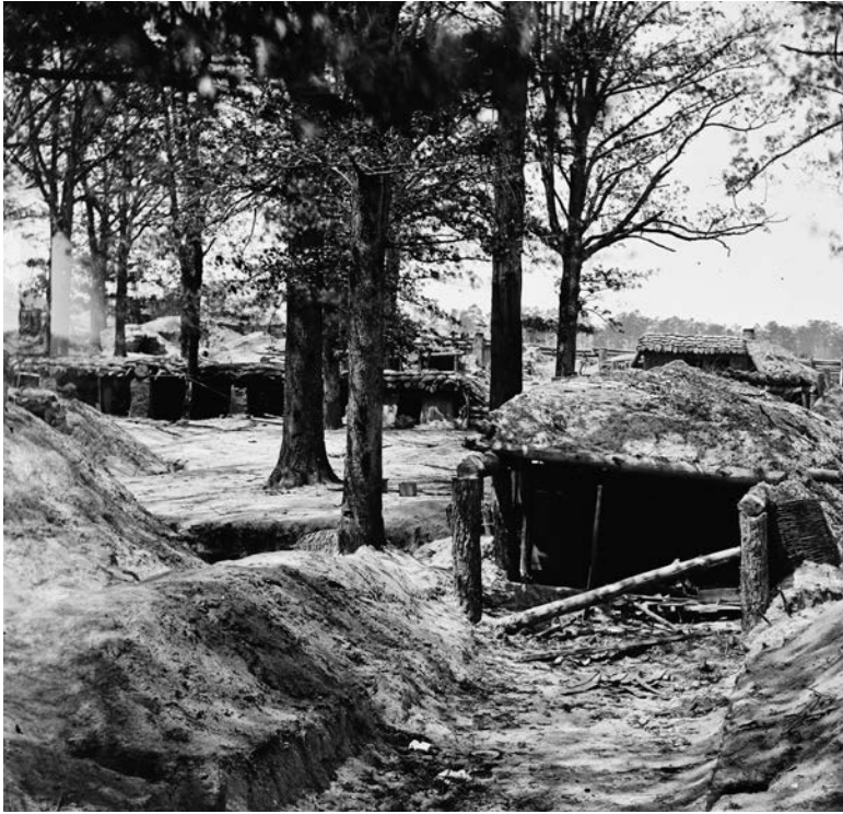
Interior of Fort Stedman (Library of Congress)
