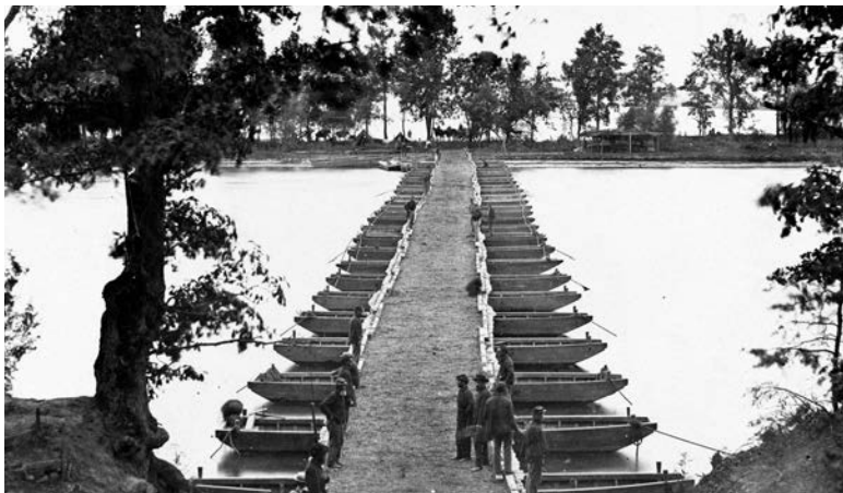
Union pontoon bridge on the James River at Deep Bottom (Library of Congress)
